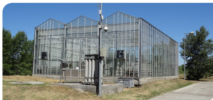
Image 1: Location of pilots, the algae glasshouse at the North Budapest wastewater treatment plant operated by Budapest Sewage Works
